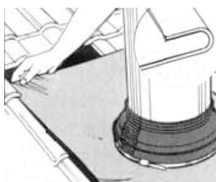
Flatten the sheet lead and form an anti-capillary fold (10mm x 2mm approx.).
