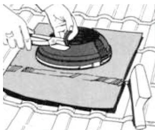
Trim the tile roof flashing cone to suit the tube size.
